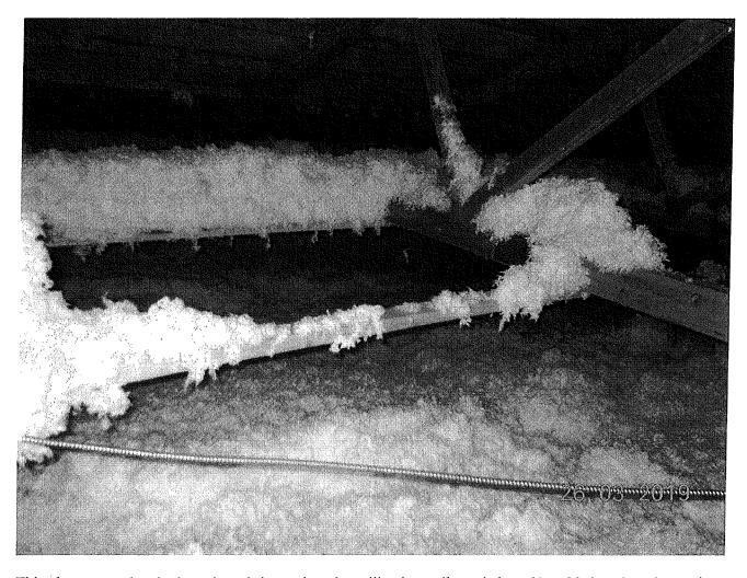
This photo was taken in the attic and shows that: the ceiling has collapsed about 3' at this location; the steel ceiling panels were not nailed to the furring strips that remain connected to the bottom chord of the truss; the depth of insulation is about 16"; separate hangers for ductwork, other than connection through the steel panel into the furring strip, are not evident.
