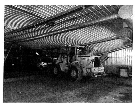
The end loader is shown holding up the steel liner panels. If the end loader were moved the ceiling would continue to collapse, The ceiling is only temporarily stabilized and the ceiling support system has little or no safety factor available to stop the failure mode.
