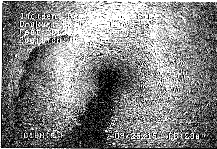
BSV - Pipe Broken: Soil Visible @ 188.8 ft.
