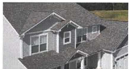
ROOFING AND VENTILATION
