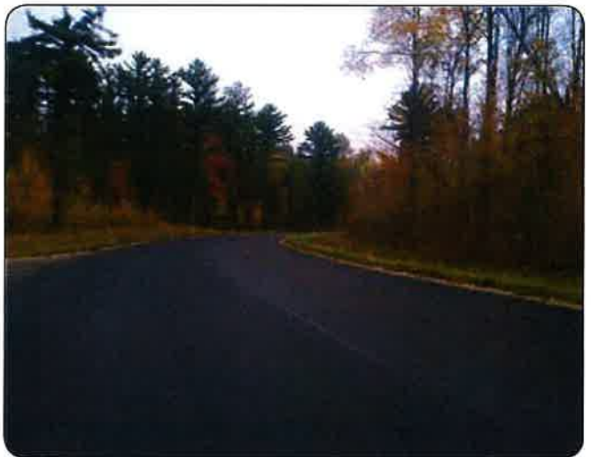
◆ Step Four: Let surface dry, broom excess sand, open project to traffic.
