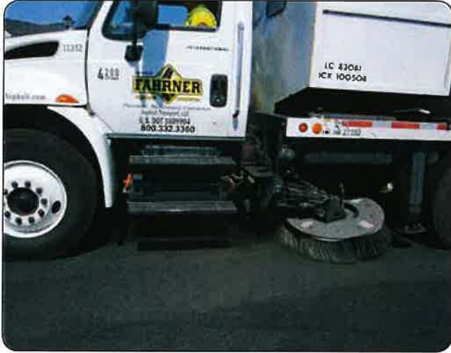
◆ Step One: Clean asphalt surface so it is free of all debris.
