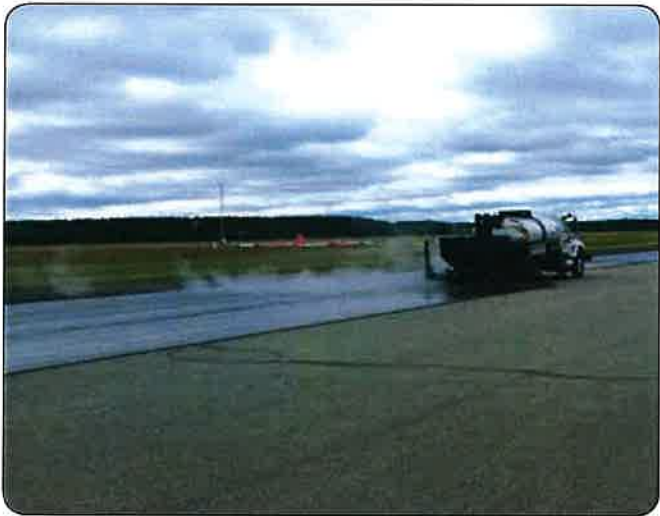
◆ Step Three: Apply GSB and sand to mainline areas.
