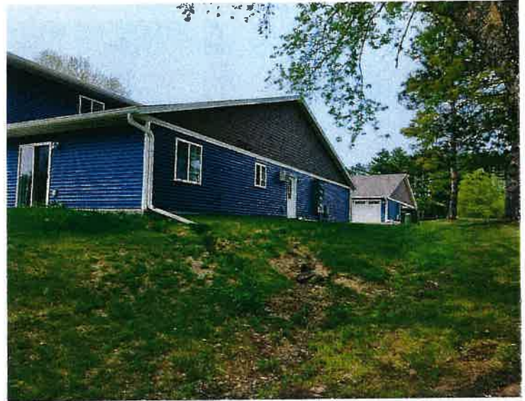
Southeast corner looking northwest
