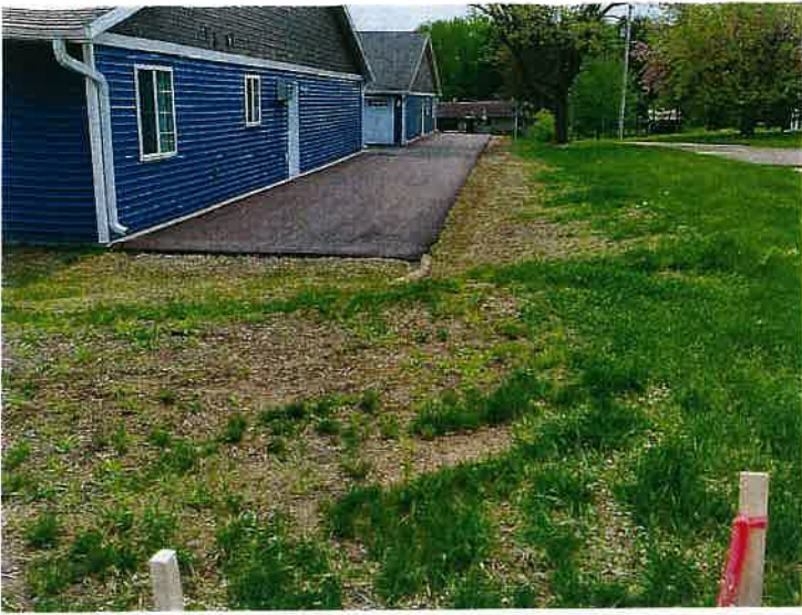
Along the back unit west side
