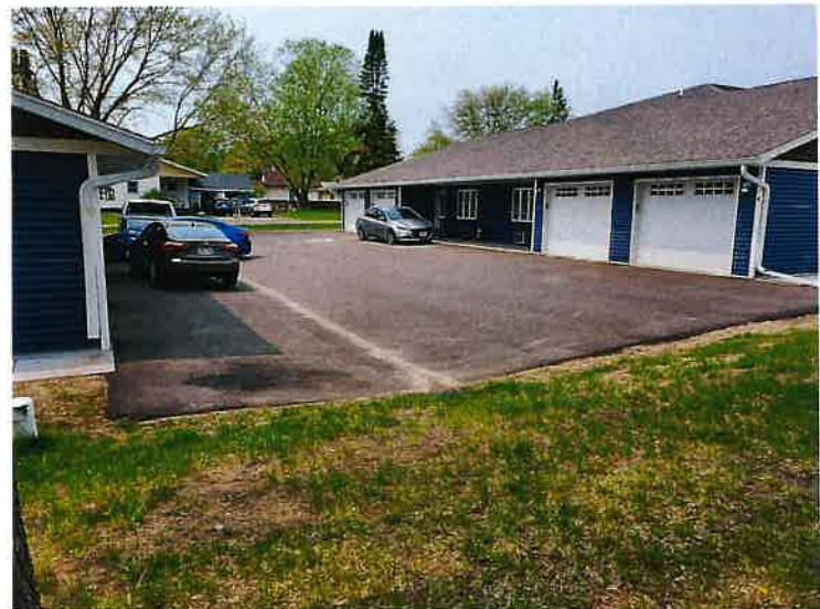
Space between the buildings facing west
