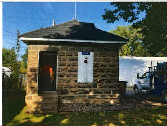
Picture Two Notes: Set up for pulling pump. Back in where service truck is
